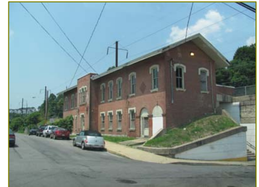
The redevelopment of the Coatesville Train Station has consistently been a priority of many different economic and transportation organizations.
